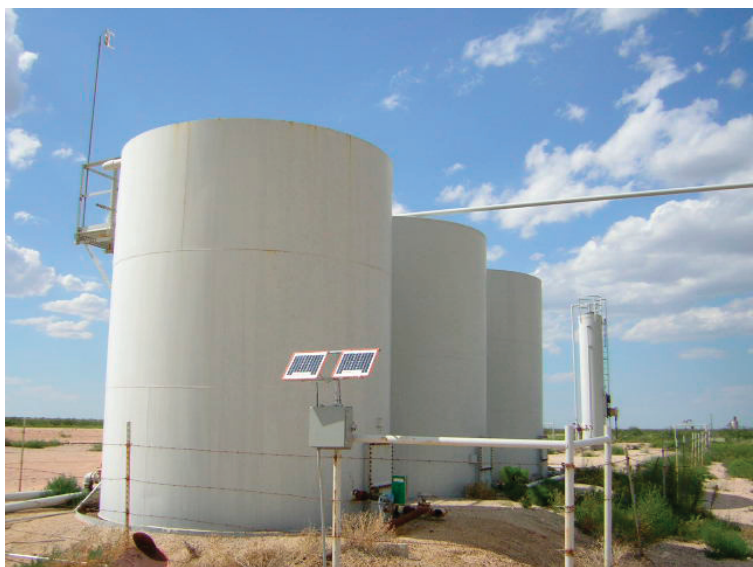
Wellkeeper continuously monitors well sites and tank batteries, allowing operators to see what's happening in real-time and over time via a Web interface.
